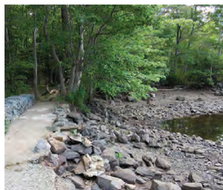
Same view as at left but here, on Sept. 10, 2020, lake level is 130 cm below top of dam, water's edge 5 meters in front of dam
