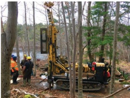
Drilling Rig at Williams Lake dam, December 2023 Photo : Cathy Vaughan
