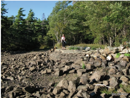
The Williams Lake dam, Sept. 2016 (Photo -Philip Howard)
